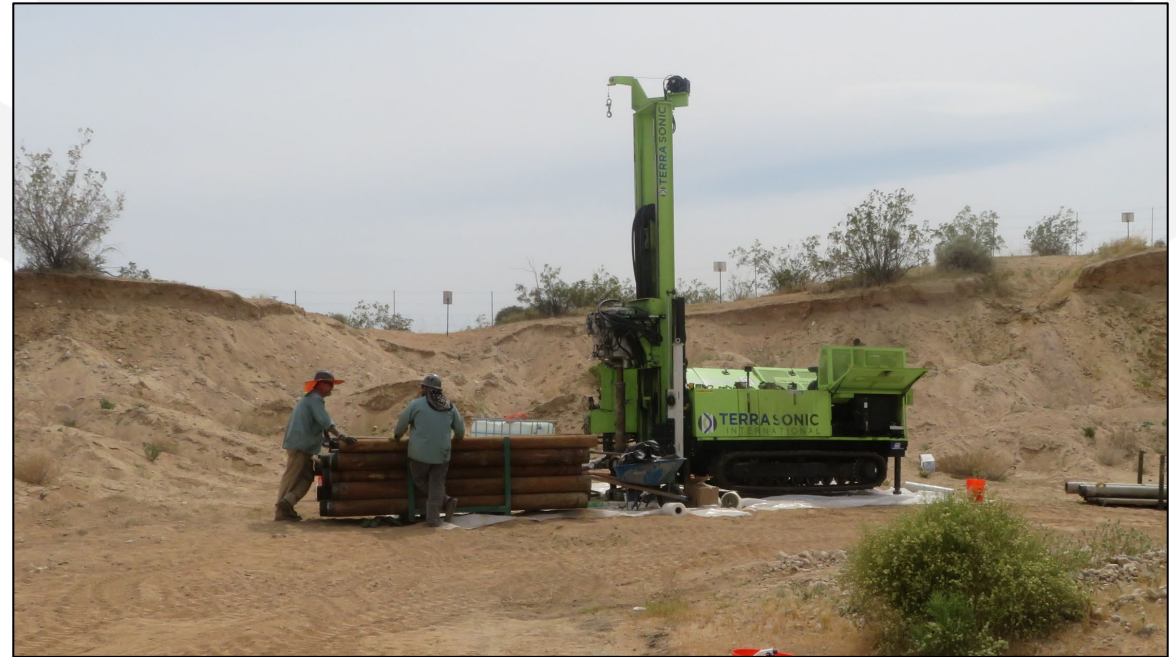
Photo of monitoring well installation
