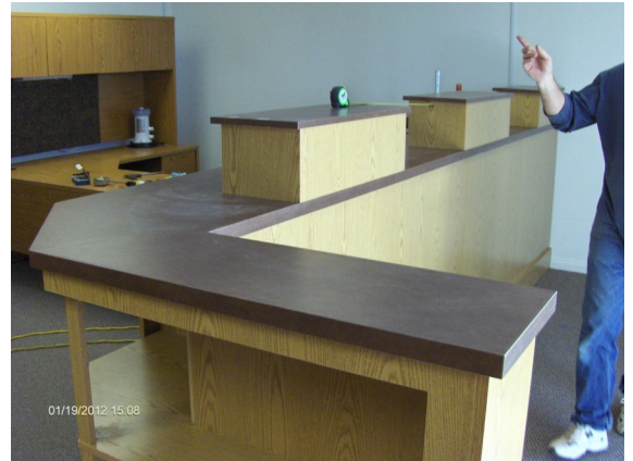
New CSD Front Counter at 26540 Vista Rd
